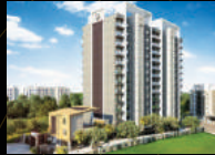
GOODWILL FABIAN PORWAL ROAD - DHANORI JUNCTION
